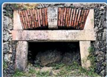
Mina do Azeche Mine Entrance
